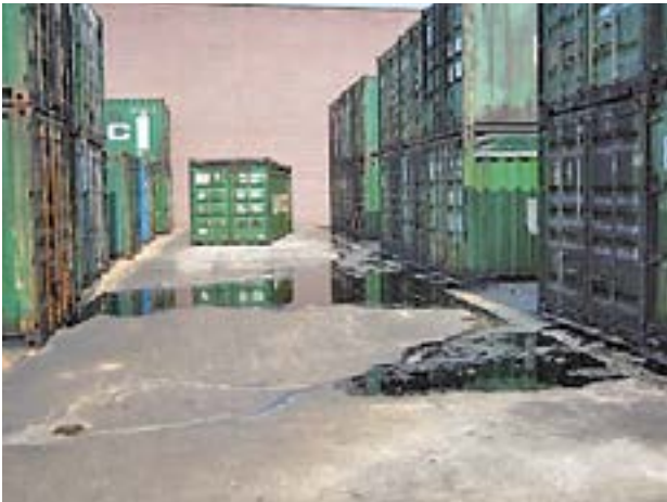
Photo: Leaking containers (source: © Courtesy of the IMPEL network)
