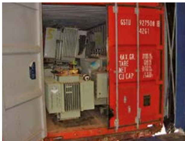
Photo: PCB containing transformers (source: © picture courtesy of the IMPEL network)
